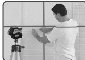
CERAMIC TILE INSTALLATION
